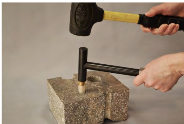
Figure 2. Installing the Vapor Pin™.
